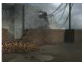
Bombed Building - 3 angles
